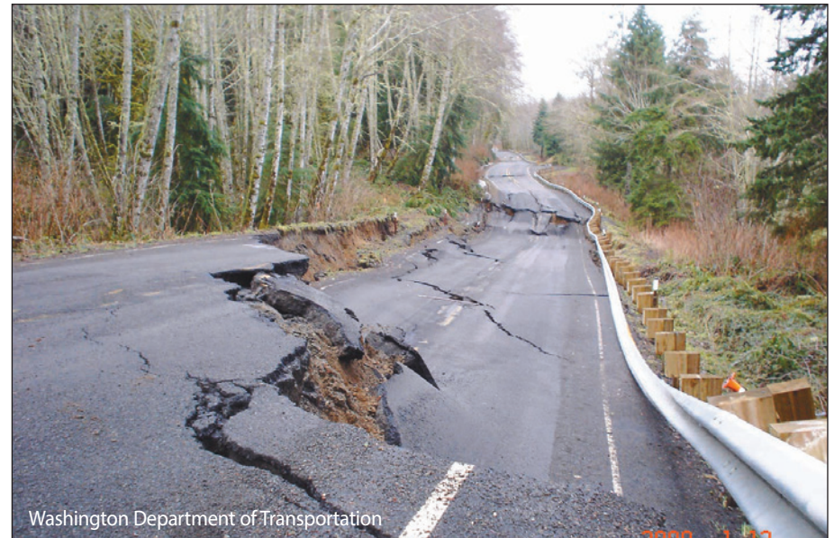
Above: In 2009, state Highway 112 sank up to 8 feet in some places after a landslide west of Joyce.
