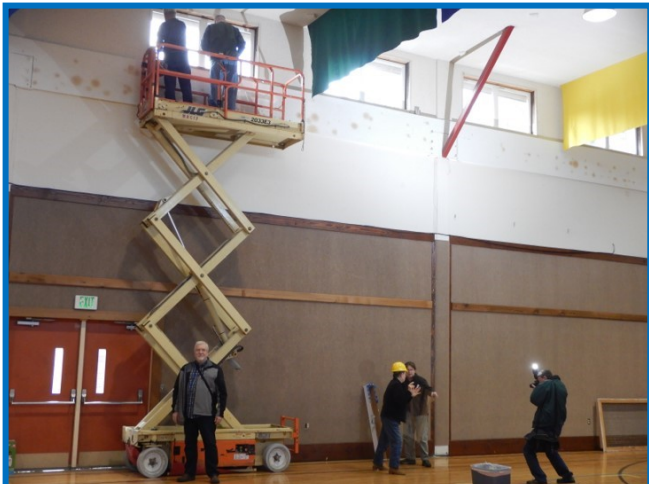
JEPP volunteers applying anti-shatter film to the shelter windows to prevent glass breakage during an earthquake.
