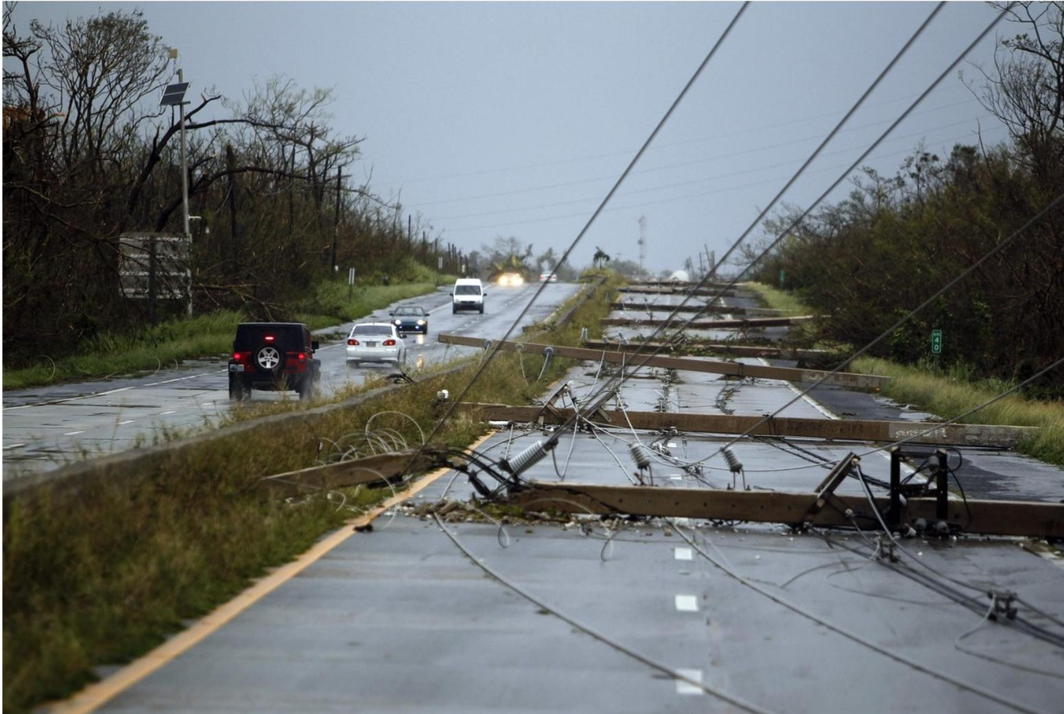
Power lines were so heavily damaged they were left where they lay and new ones strung. Picture is 2 days after the event.
